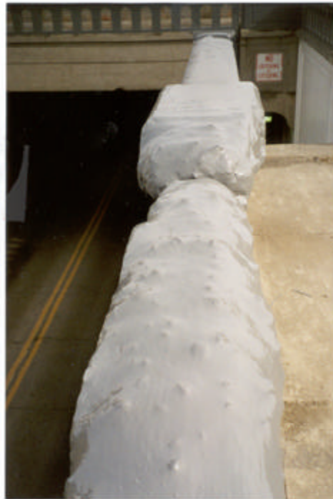
ENCAPSULATING DETERIORATING CONCRETE BRIDGE WITH POLYSHIELD SS-100™
