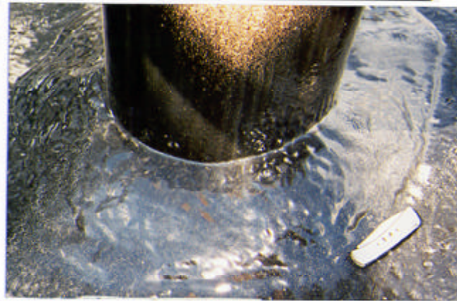
USING POLYSHIELD SS-100™ AND POLYURETHANE FOAM ON GEOTEXTILE FABRIC TO REPAIR AND EXTEND URETHANE LINER
